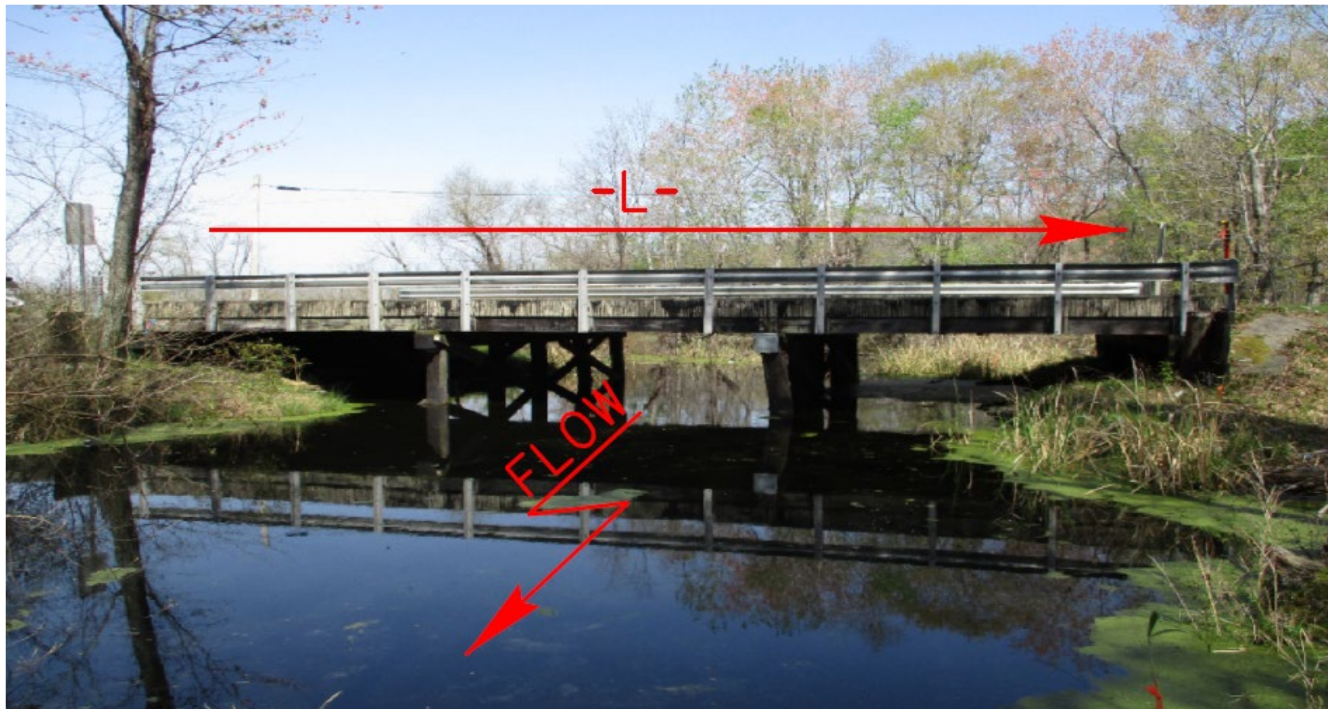
Bridge No. 18 on -L- (SR 1510) over Paddy's Delight Creek
